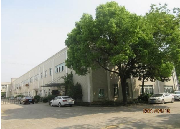
Factory building-production & office
