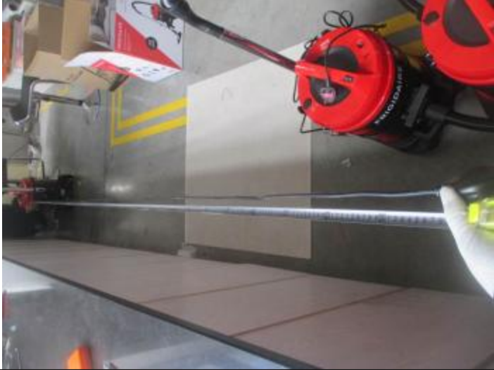
IMG_219 Length of power cord check
